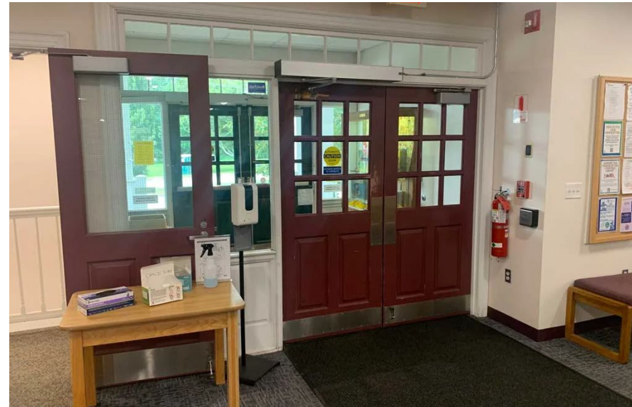
Entrance hard to navigate with wheelchairs / walkers / strollers
