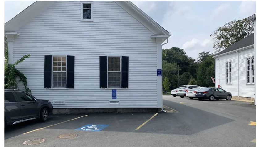
Single dedicated handicapped spot in parking lot
